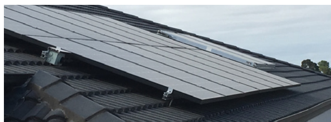
Installed a 4kw solar system
