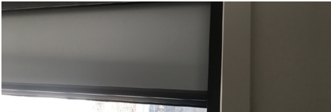
In many rooms window sizes were reduced and screen away blinds installed to block radiant heat from the sun.
